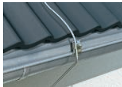
Conductor, connected with gutter clamp
