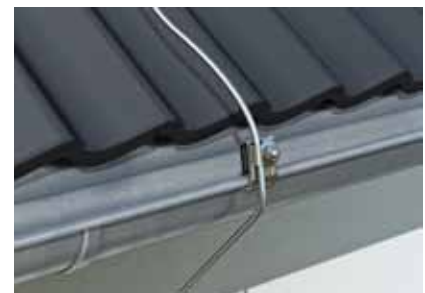
Conductor, connected with gutter clamp
