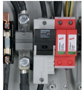
Fig. 9.18.1.3 Modular surge arrester Type 2 DEHNguard S PV SCI 600 for use in earthed d.c. systems
