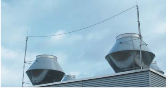
Fig. 5.2.4.2.3a Fan with air-termination rod and spanned cable
