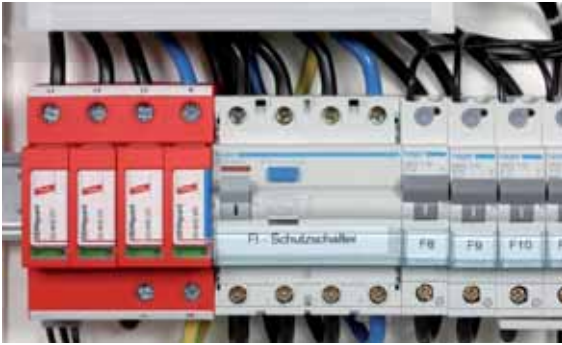
Fig. 7.7.2.3 Multi-pole surge arrester DEHNGuard M TT
