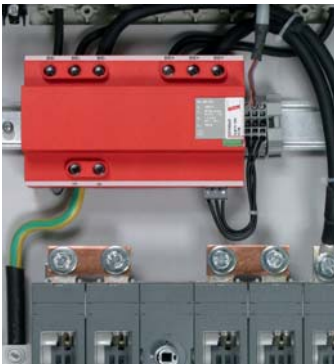
Fig. 9.18.1.1 Combined arrester Type 1, DEHNlimit PV 1000 V2 FM, to protect photovoltaic inverters from surges also in case of direct lightning strikes
