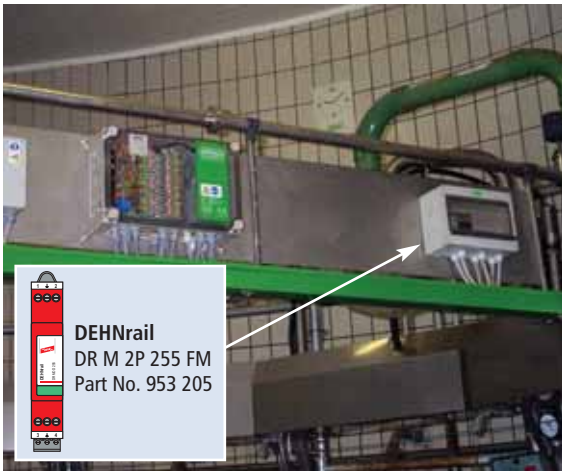
Fig. 9.6.5 Electrical milking system with control box
