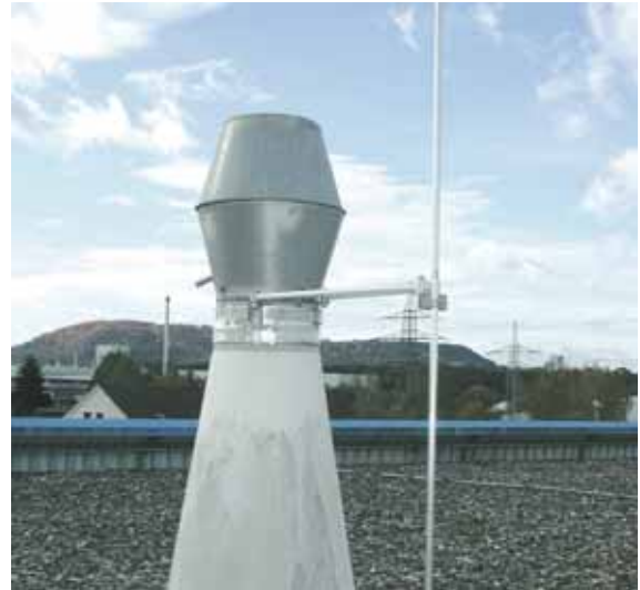
Fig. 5.1.8.3 Air-termination rod with distance holder
