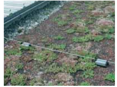
Fig. 5.1.7.3 Conductor leading on the covering layer
