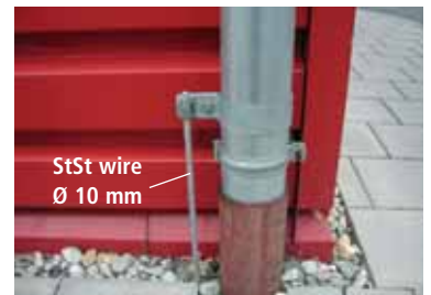
Fig. 5.2.2.1.4 Earthed downpipe
