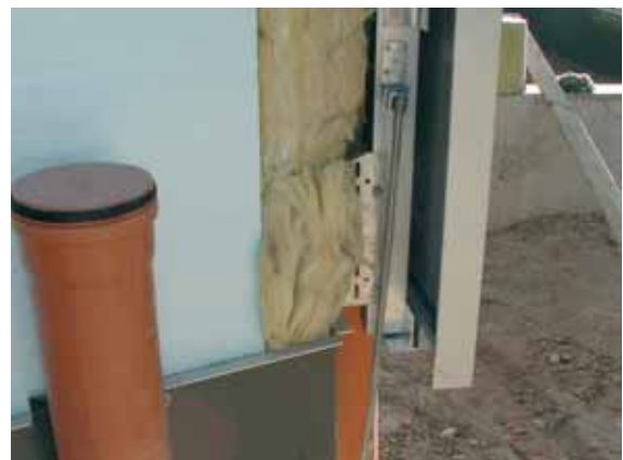
Fig. 5.2.2.2.3 Earth connection of a metal facade
