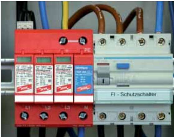
Fig. 7.8.1.2 DEHNGuard TT H LI – Multi-pole surge arrester with service life indication
