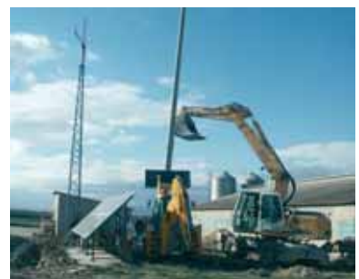
Fig. 5.1.8.9 Installation of a steel telescopic lightning protection mast
