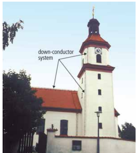
Fig. 5.1.9.1 Installing the down-conductor system at a steeple
