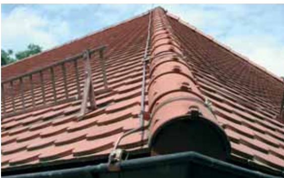
Fig. 5.1.1.18 Gable roof with conductor holder
