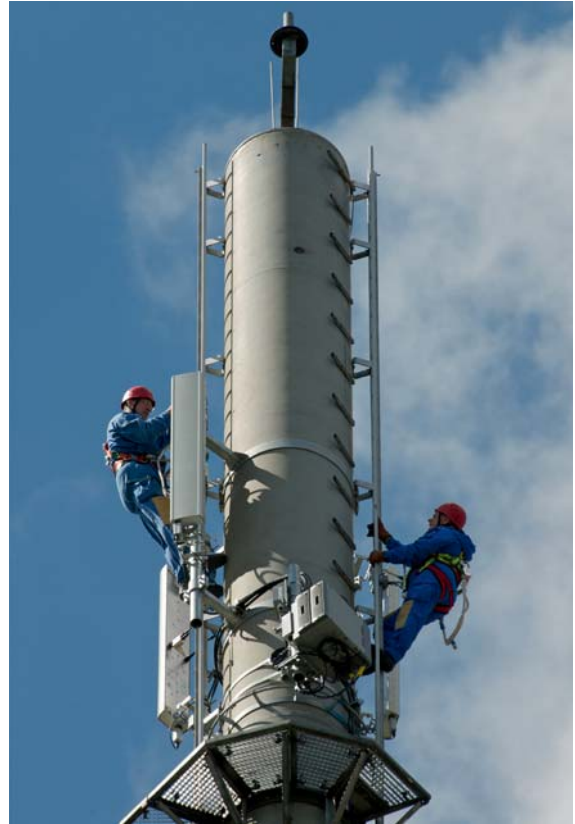
Fig. 9.17.1 T-Mobile (Brandenburg), LTE (Long Term Evolution) configuration; Source: obs/Deutsche Telekom AG
