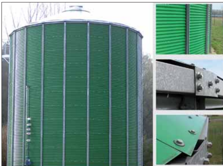
Fig. 9.3.6 Fermenter out of screwed sheet metal
