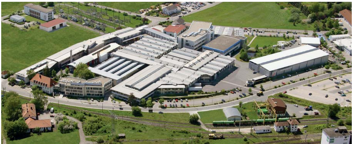
Aerial photo of DEHN + SÖHNE
