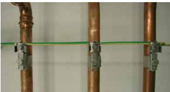
Fig. 6.1.6 Equipotential bonding with straight-through connection
