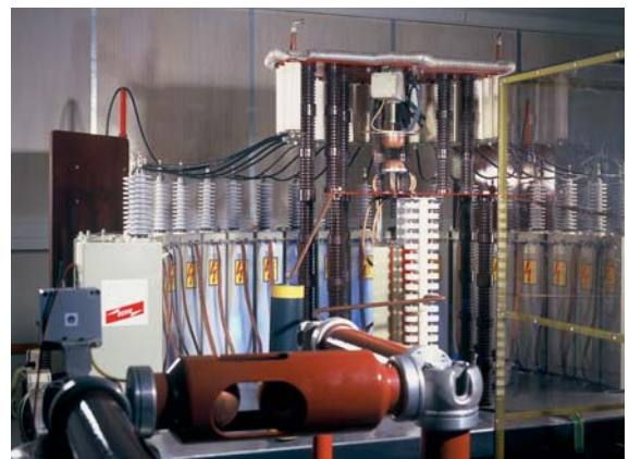
Fig. 9.16.1 Impulse current laboratory DEHN + SÖHNE – Max. lightning impulse current 200 kA, wave form 10/350 \mu s
