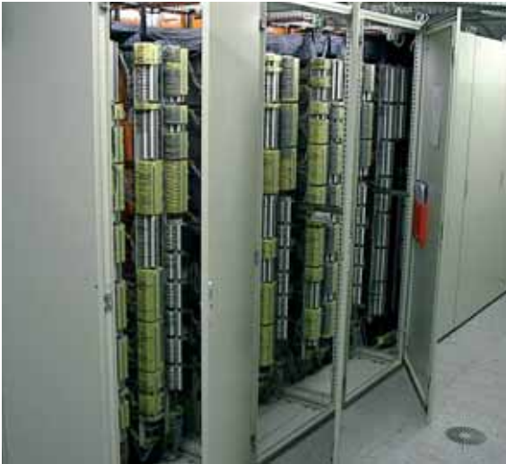
Fig. 9.4.7 DCO ME 24 surge protective device installed into a switchgear cabinet for protection of the complete measuring and control system
