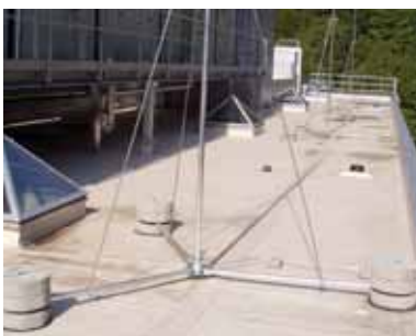
Fig. 5.1.8.7 Isolated air-termination system for roof-mounted structures
