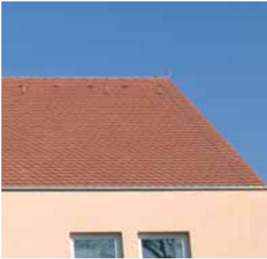
Fig. 5.1.2.1 Air-termination system on a gable roof
