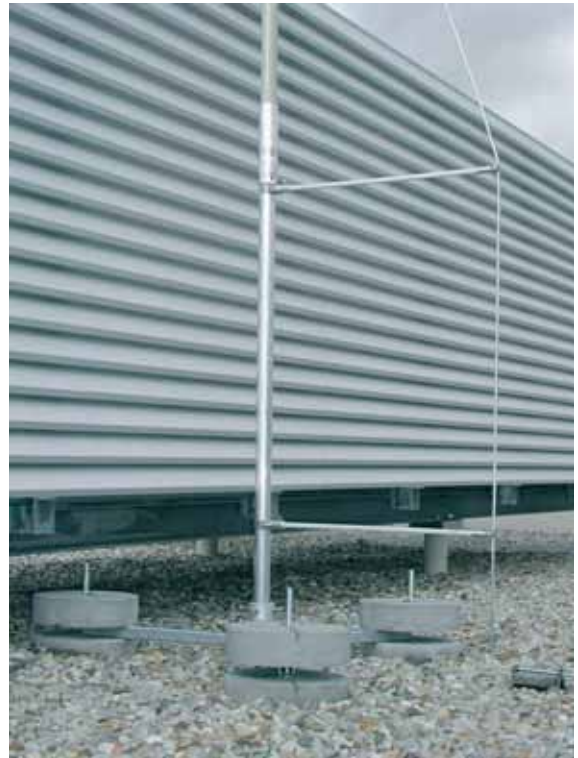
Fig. 5.1.8.11 Tripod support for self-supporting insulating pipes
