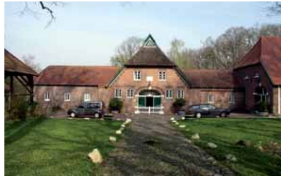
Fig. 5.1.5.4 Historical farmhouse with external lightning protection (Ref. Photo: Hans Thormählen GmbH & Co.KG)
