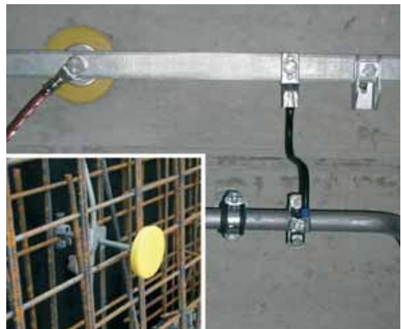
Fig. 5.5.2.8 Fixed earthing terminal
