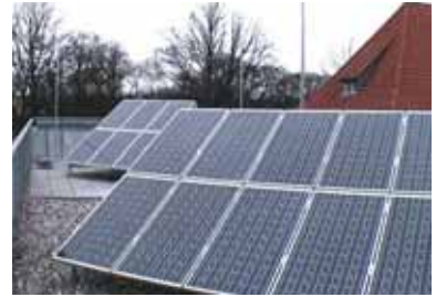
Fig. 5.1.8.6 Isolated air-termination system for photovoltaic system
