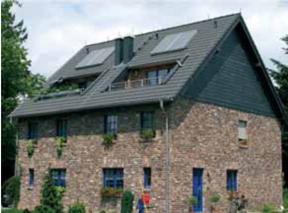
Fig. 5.1.2.4 Building with photovoltaic system Ref.: Wettingfeld Lightning Protection, Krefeld, Germany
