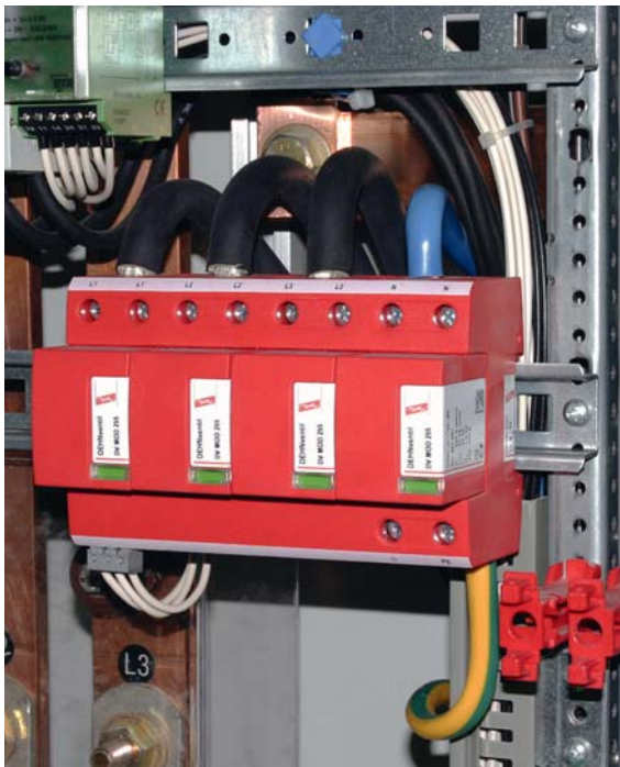
Fig. 6.2.2 DEHNventil combined lightning and surge arrester for installation in conformity with the lightning protection zones concept at the boundaries O_A - 2
