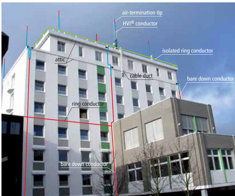
Fig. 5.2.4.3.4 Total view on a newly installed external lightning protection system
