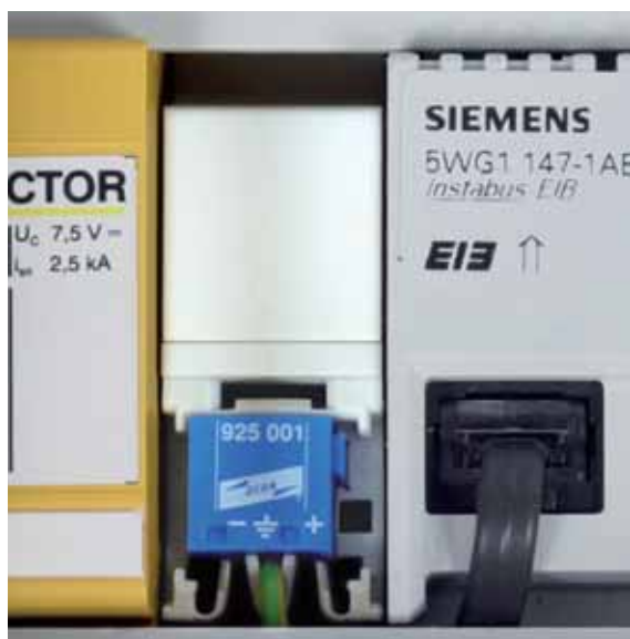
Fig. 9.10.1 Application of the BUStector (Part No. 925 001)
