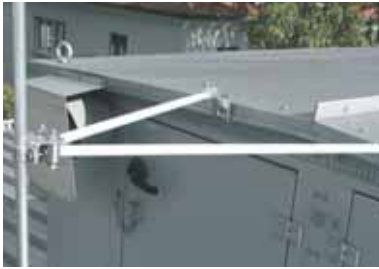
Fig. 5.1.8.4 Angled support for air-termination rods
