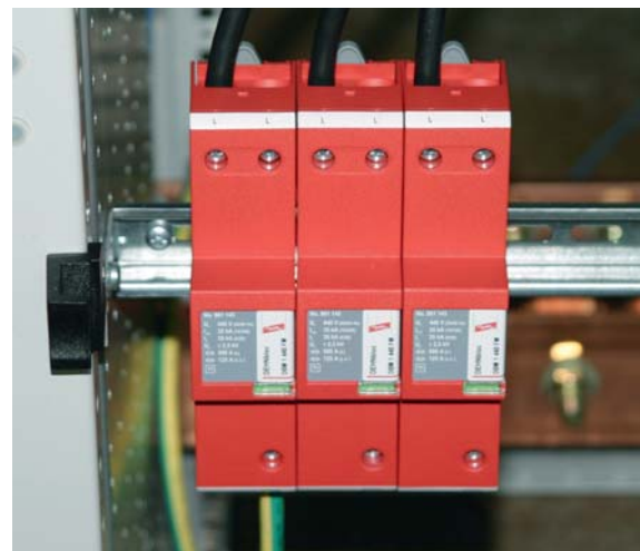
Fig. 9.16.4 Application of DEHNbloc Maxi coordinated lightning current arrester for 400/690 V TN-C systems
