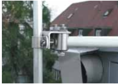
Fig. 5.1.8.5 Supporting element for the air-termination rod
