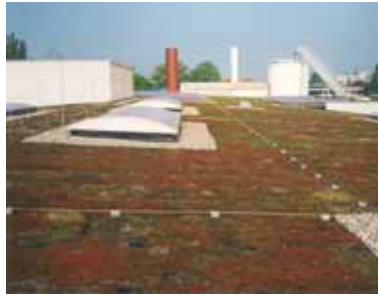
Fig. 5.1.7.2 Air-termination system on a green roof
