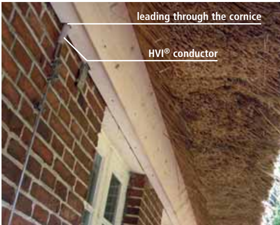
Fig. 5.1.5.7 HVI conductor led through the cornice plank
